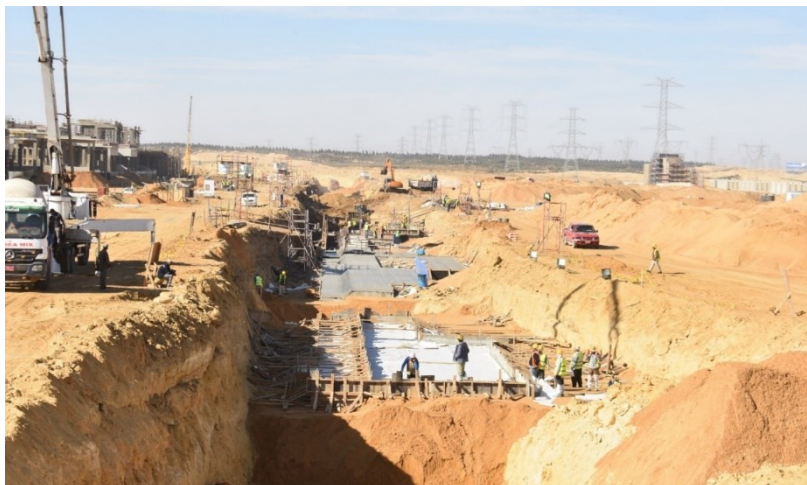
Figure 6: Utility Tunnel Construction "New capital of Egypt"
