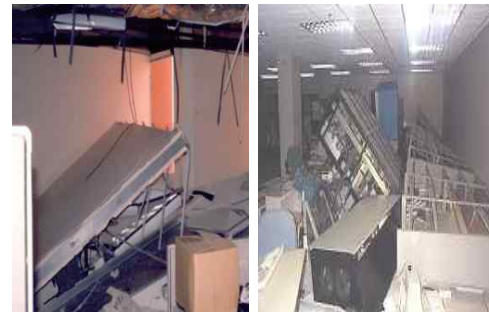
Fig. 1. Earthquake damage of the nonstructural components
